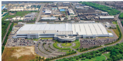
DENSO MANUFACTURING KITAKYUSHU CO., LTD.
