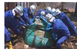
Associates carrying out recovery work at disaster-affected areas of the Great East Japan Earthquake
