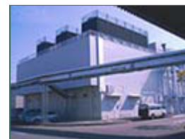
Co-generation facilities at Daian Plant
