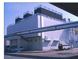
Co-generation facilities at Daian Plant
