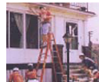
Volunteer activity repairing damaged houses of the socially disadvantaged (DIAM, U.S.A.)
