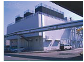
Co-generation facilities at Daian Plant
