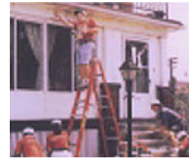
Volunteer activity repairing damaged houses of the socially disadvantaged (DIAM, U.S.A.)
