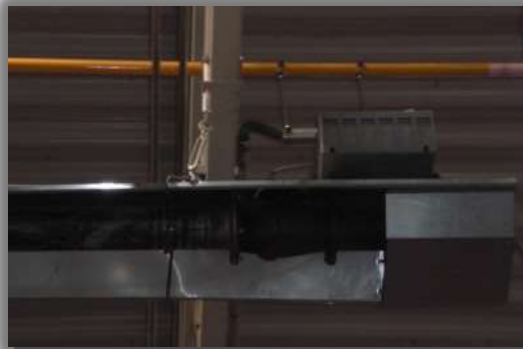
Burner of one of the radiating pipes
