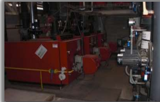
DNBA Boiler Room
