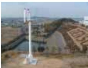
Wind-power generator for external lighting at the Zenmyo Plant in Japan
