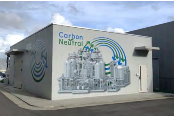
Fig. 6 Demonstration plant appearance
