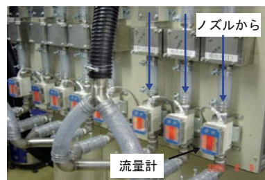
Fig. 13 Installation states of Roots blowers and flowmeters
