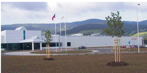
DENSO Manufacturing Czech s.r.o.
